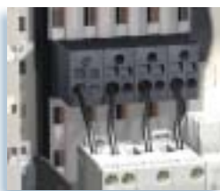
Tap-off terminals and supply of switchgear
